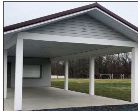
Restroom, Pavilion & Concession Stand at Valley Road Park Colby Lupfer Eagle Scout Project
